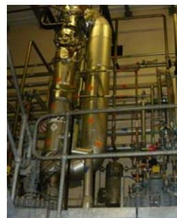
*“Colour coding process plant for varying levels of contamination to assist decommissioning and decontamination”*
